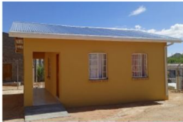
Classroom built at Feetjeland
